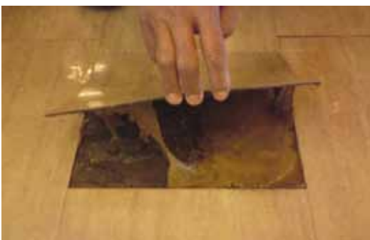
Flooring failures
