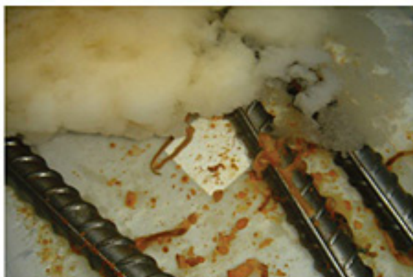
■ Example of corrosion inhibition
