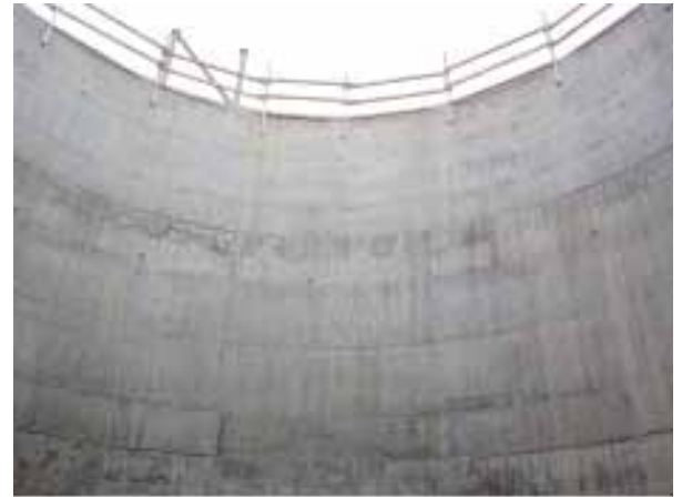
Pit wall cast with Hycrete W1000 admixture
