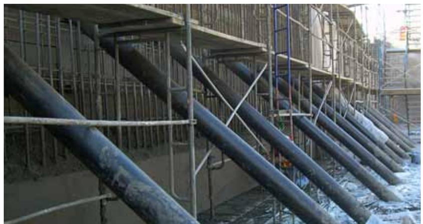
Simple waterproofing for shotcrete walls using Hycrete System W. No separate trade. No surface preparation. No tricky detailing around raking props or tie-backs. No problems caused by waterproofing being damaged by shotcrete pressure. No finger pointing.
