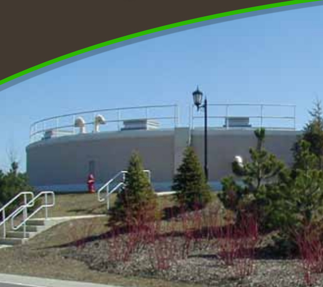
Toll Brothers, The Woods of South Barrington Community, Potable Water Tank
