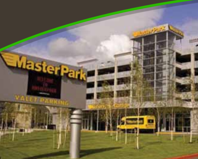
MasterPark Garage, SeaTac, WA
