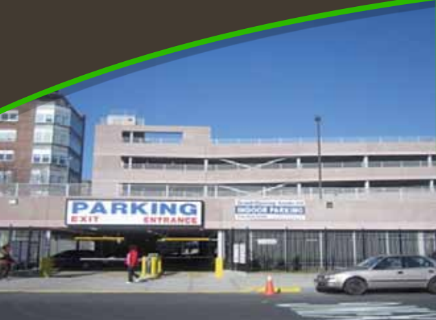
Kings County Hospital Parking Garage, Brooklyn, NY
