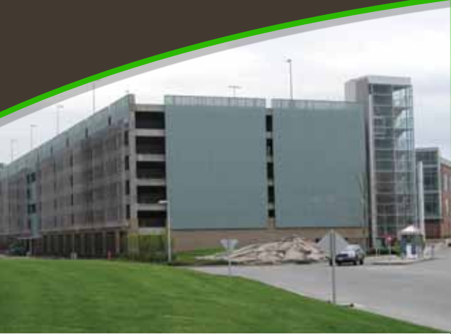
Amgen Parking Garage, Seattle, WA
